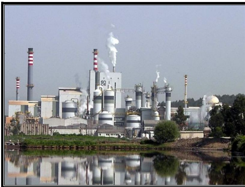
Figure E5.1-16: ENCE Mill Operating in Spain
